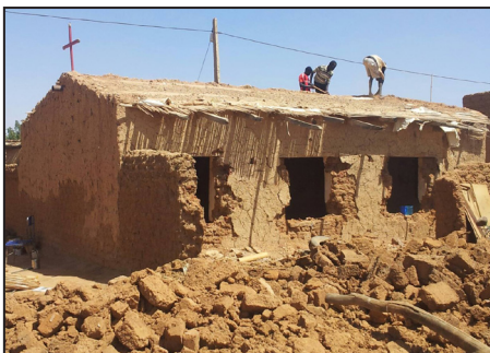
Workers tear down a church building in Omdurman, Sudan, in 2014. (Photo: Morning Star News )
